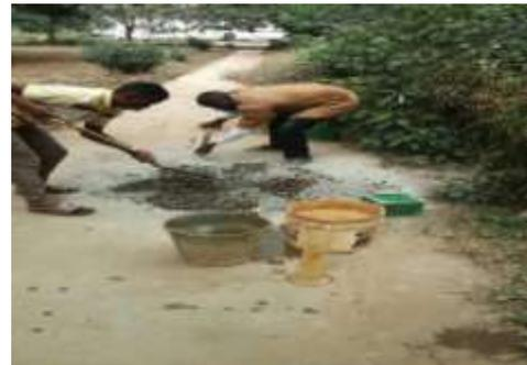
**Fig. 8. Mixing of concrete**
