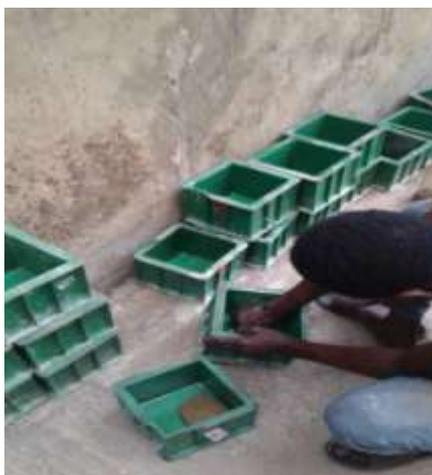
Fig. 1. Lubricating of moulds
