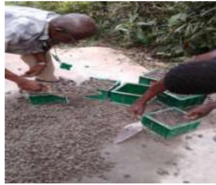
**Fig. 4. Placing the mixed concrete into the Moulds**
